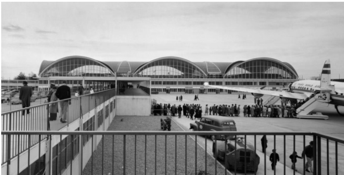
The pioneering thin-shell concrete structure of St Louis Lambert International Airport
